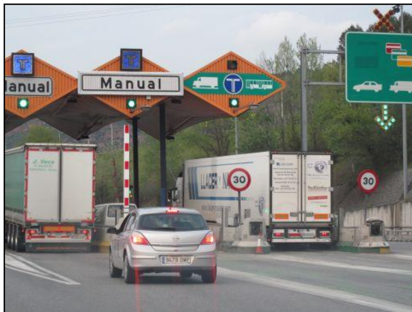
Example of a VIA-T station
